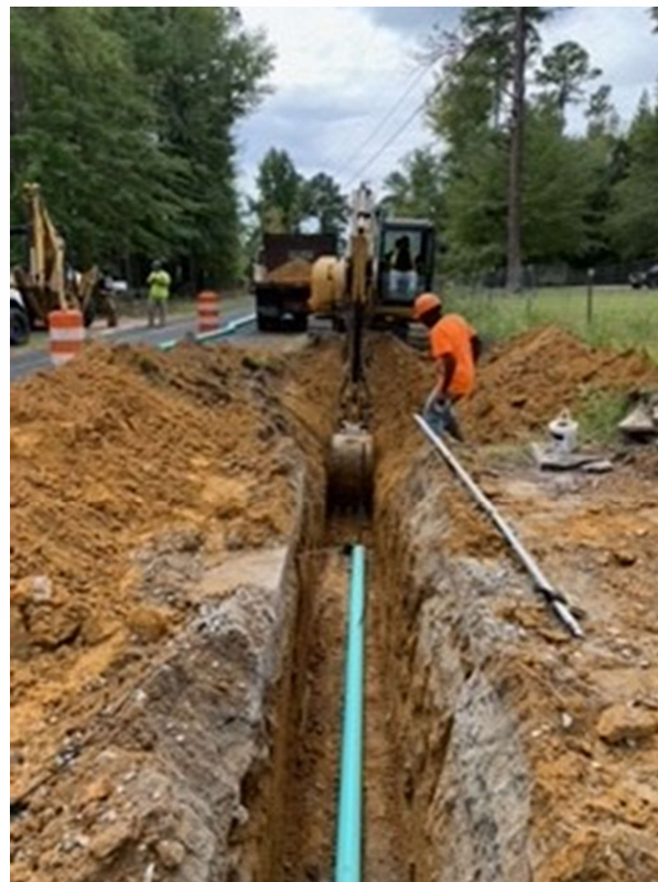
Photo 4: Force main install
