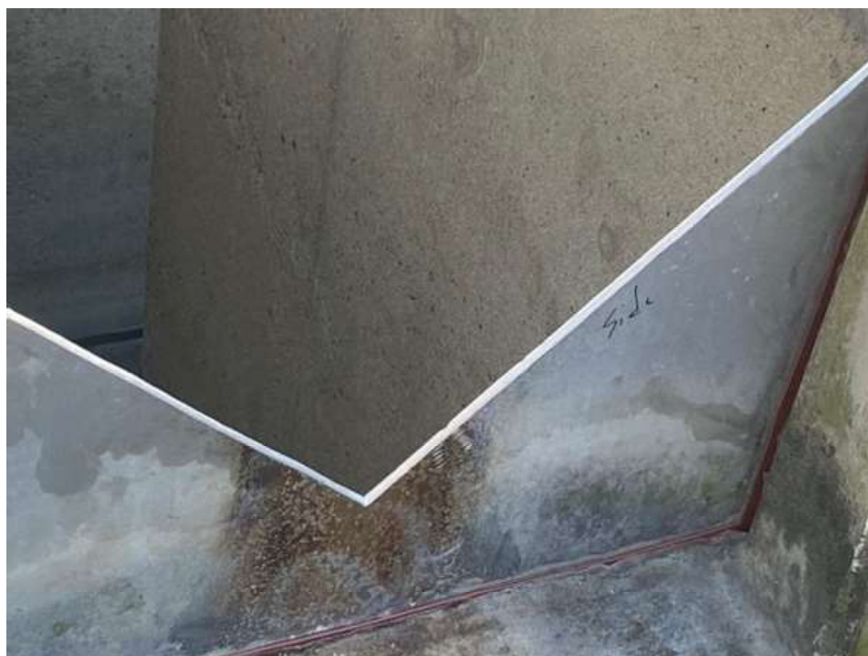
Photo 2: Weir install
