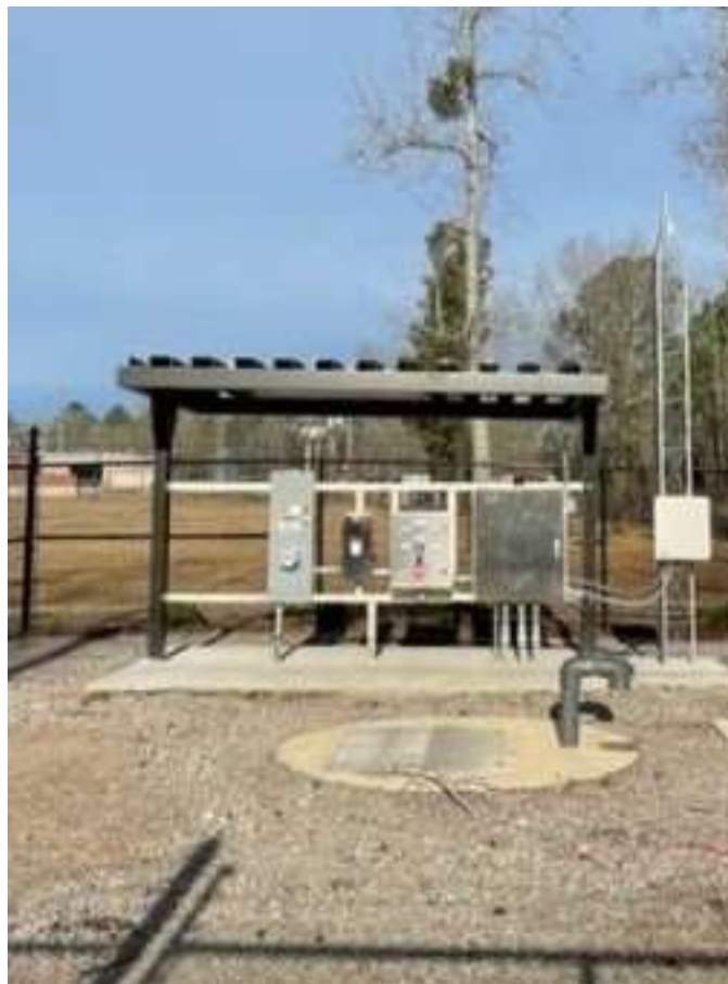
Photo 3: Control panel install
