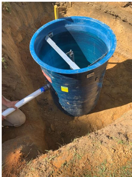
Photo 4: Grinder pump install
