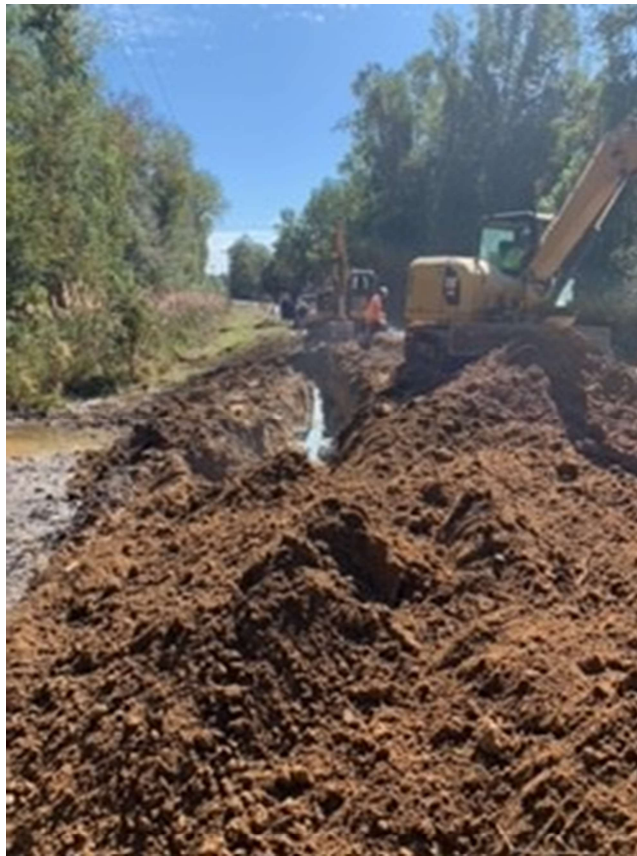
Photo 4: Force main install
