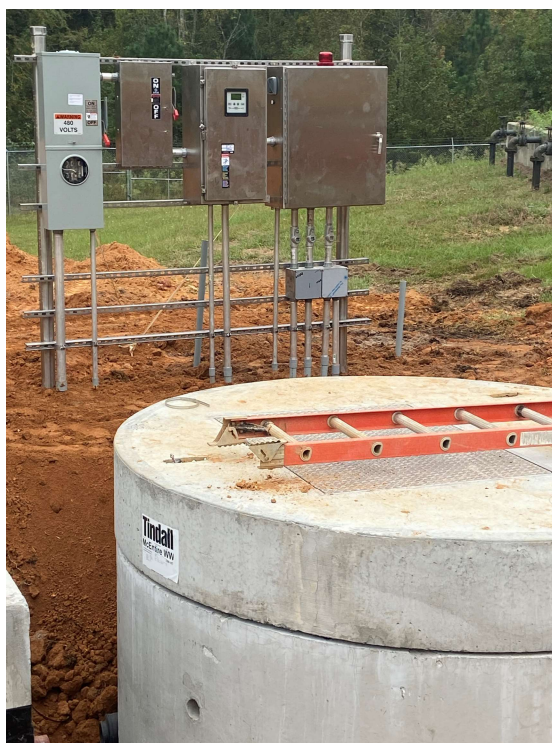
Photo 2: Wet-well install
