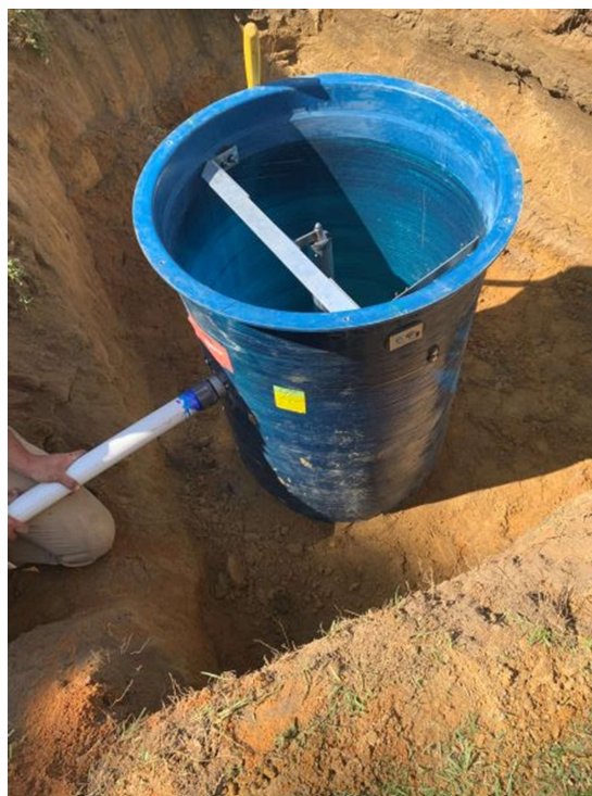
Photo 4: Grinder pump install
