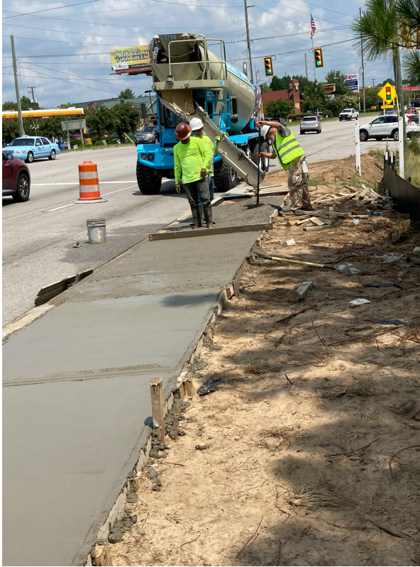
Concrete Pouring at Clemson Road Sidewalk
