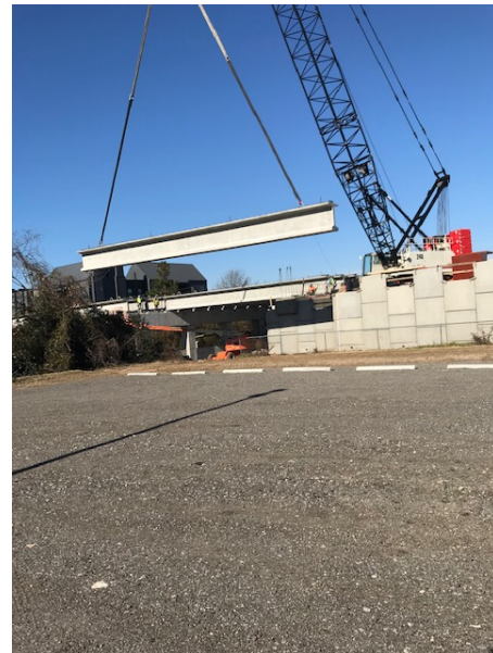
Greene St. Bridge Installation
