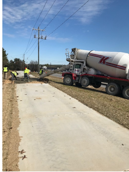
Polo Rd. Sidewalk Installation
