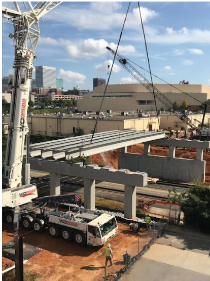
Innovista – Greene St. II Girder Installation
