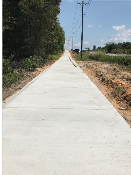
Polo Rd. SUP Concrete Installation
