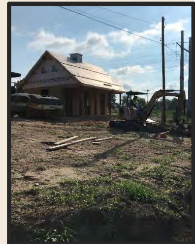
Progress on the public restroom along the Three Rivers Greenway.
