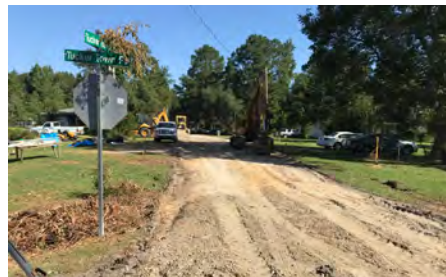
Tucker Town Court dirt road paving
