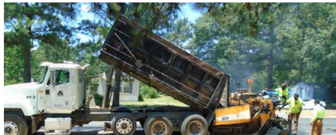
Joster Street dirt road paving
