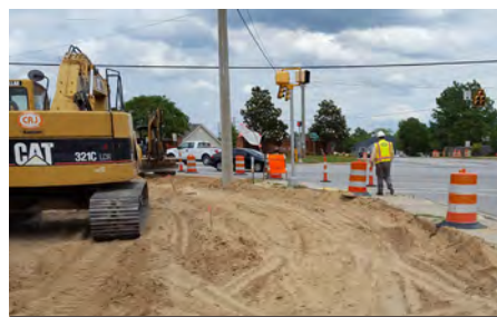
North Springs/Clemson Road Intersection
