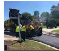
Cove View Drive Resurfacing Project
