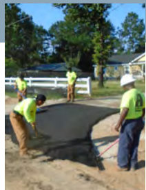
Joster Street dirt road paving
