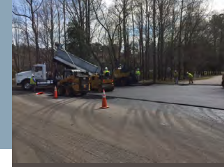
Repaving Finley Road
