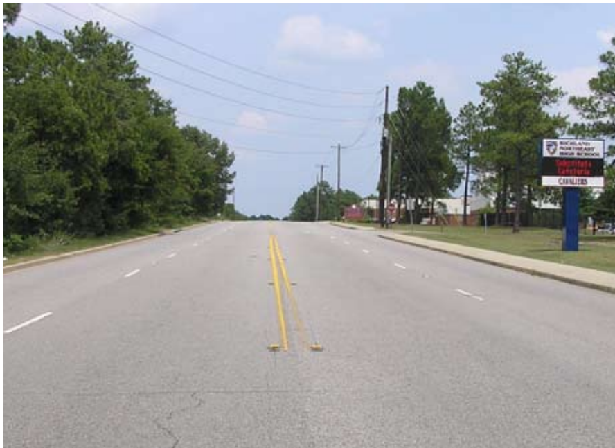
Photo of existing Brookfield Road street section, which includes 4 12-foot lanes, 1 foot gutters, and a 5-foot sidewalk on the south side (high school side) only.
