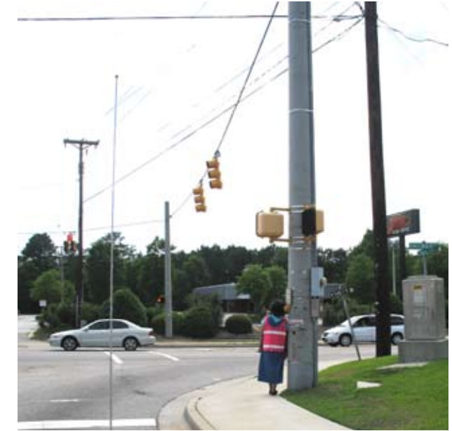
Existing intersection as seen from O'Neil Court
