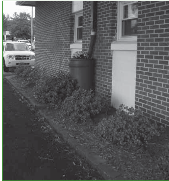
Rooftop runoff captured by a rain barrel
