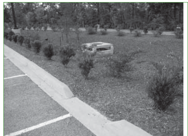
Parking lot runoff treated by bioretention
