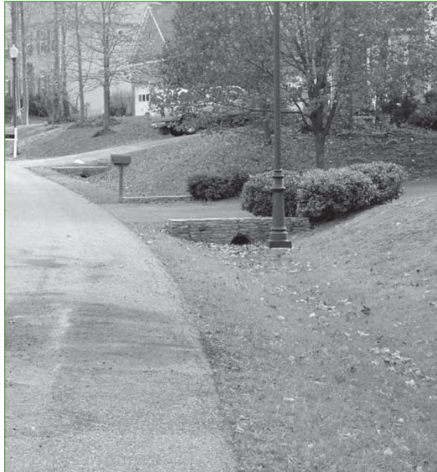
Vegetated open channel along residential street
