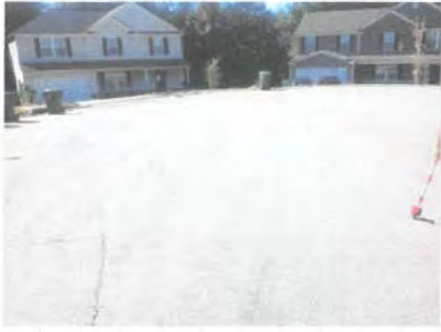
Cul de sac 96x80 alligator and reflective cracking. 87 ft curb damaged binder course surface course not installed
