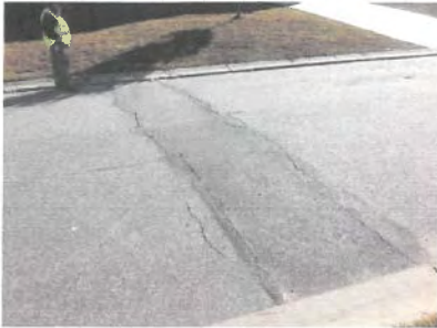
30 ft curb damage in front of house 333 Blythe Creek drive. An additional 30ft curb damage across street Also a utility crossing road failure of 12x24
