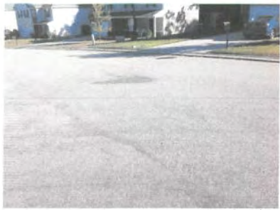
60x24 longitudinal cracking and reflective at intersection of broken arrow ct and Blythe creek dr
